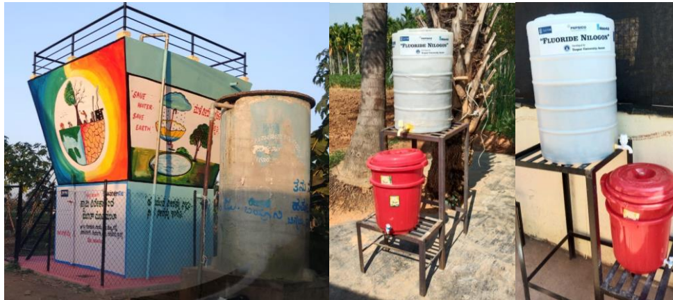
Fig. 2.iii.c. Fluoride-contaminated community water supply scheme of Gangabhairappanpalya village (left) and two of the 35 Fluoride Nilogon filters of 21 L capacity.
