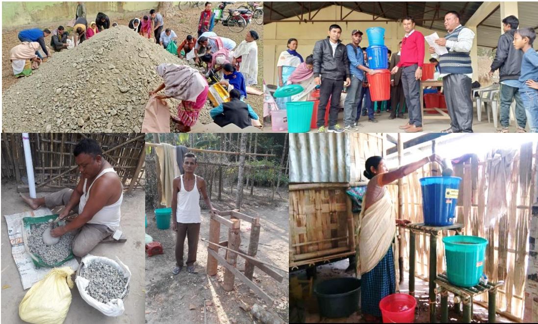
Fig. 2.v.c.1. Spontaneous involvement of villagers in installation of filters at Japarajan, Deopani, Karbi Anglong district, Assam
